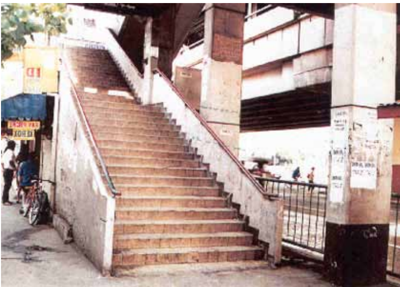
Illustration 12 34 steps leading to a terminal station of the Light Rail Transit (LRT), but with no elevator. Currently, the newly constructed terminals are now provided either with an elevator or an escalator.
