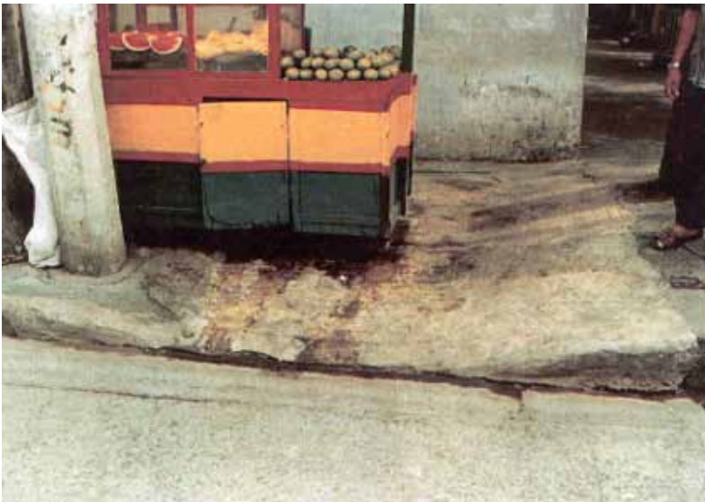
Illustration 10 A complying curb cut-out but the passage is blocked by a vendor's fruit cart.
