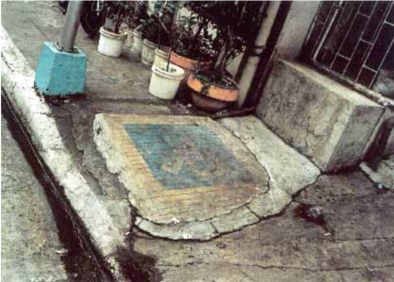
Illustration 8 A complying curb cut-out but leads to a narrow sidewalk, because of obstructions, along the passageway, such as, a light post and several potted plants.
