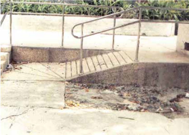
Illustration 14 A steep ramp with a 2-level handrail on one side. The slope gradient of the ramp is equal to the run of the 4 steps.
