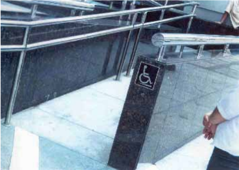
Illustration 20 An L-shape ramp with conforming ramp gradient, and innovated handrail design. As shown, there is a 2-level handrail on one side and a granite with handrail on the other side. Design innovations on ramps and handrails, have developed.
