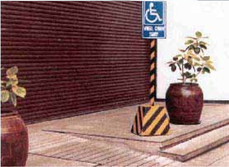
Illustration 21 A loading/unloading, rear entrance of a building, wherein it indicates that ramps are not located only at the main entrance, but also at the rear entrance of the building.
