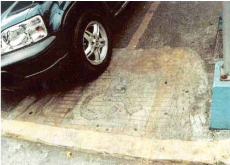
Illustration 9 A complying curb cut-out but the passage is blocked by a car.
