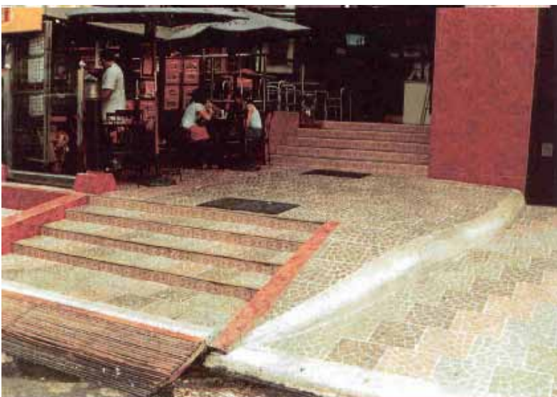
Illustration 13 9 steps leading to a restaurant, but with no ramp. 4 steps leading to an outdoor dining, and another 5 steps leading to the main doorway entrance.
