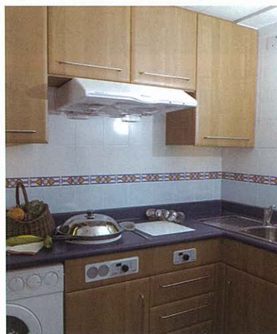
Fig 6. Electric induction cooking plates installed to reduce the fire risks brought by naked fire.
