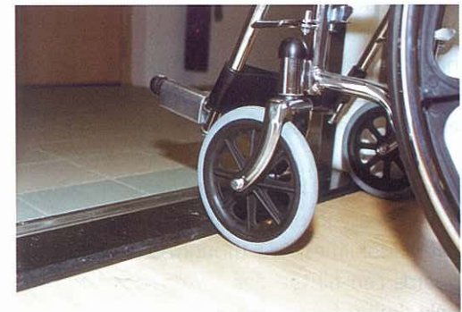
Bevelled edges are essential for the wheels of the wheelchair to glide over the threshold.
