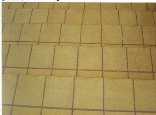
Homogenous colour treads make level differences indistinguishable.
