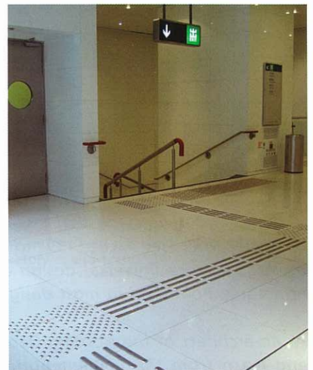
Fig 7. Provide clear signage and tactile path.
