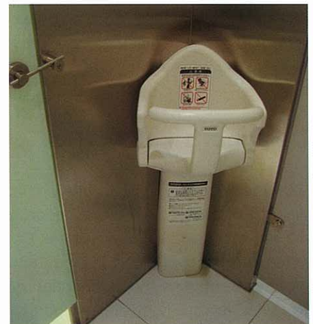
Fig 8. Provide baby seat inside toilet cubicle. The addition of signage would enhance access.
